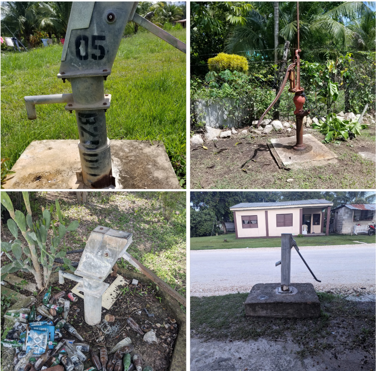
Figure 2.4: Example of community handpumps
