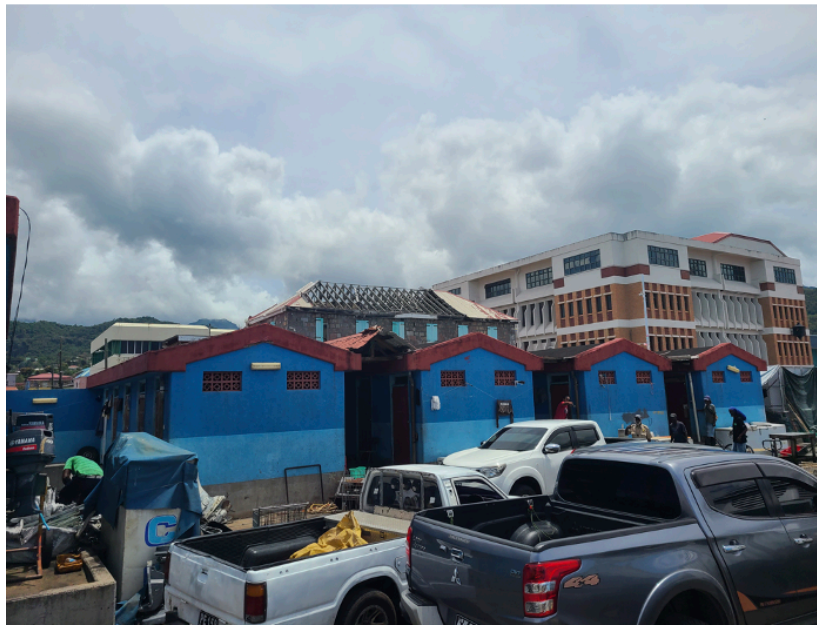
Figure N. Roseau Fisheries Complex, Mechanical Workshop Buildings
