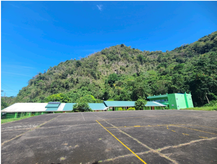
Figure O. DCHS One-storey (left) and Two-storey buildings (right)
