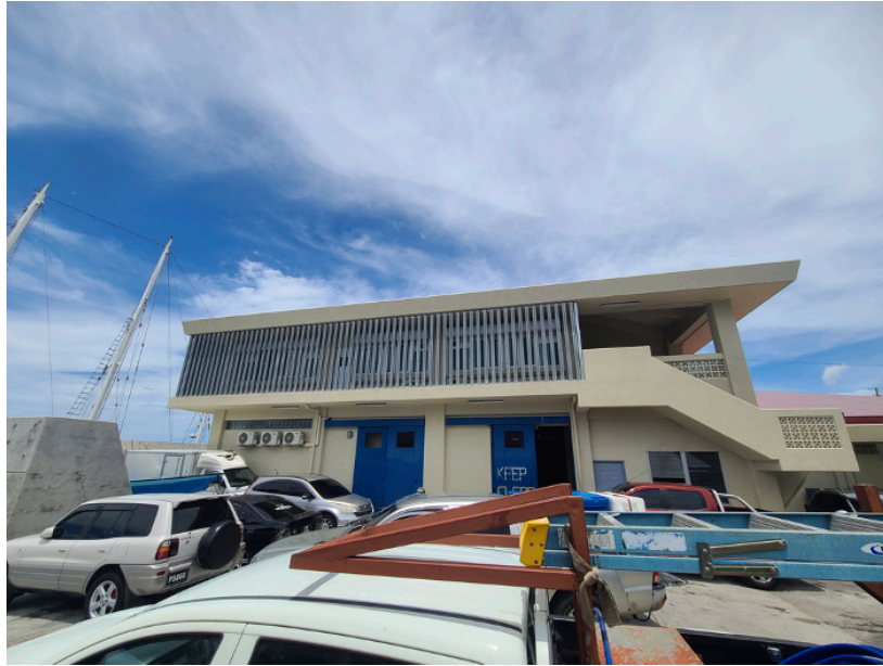
Figure M. Roseau Fisheries Complex, Main Office/Industrial Building
