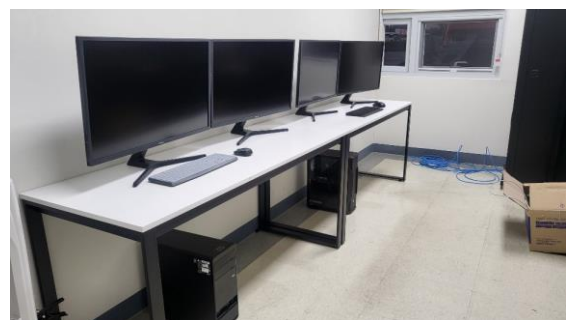
Operator Terminal (Office)
