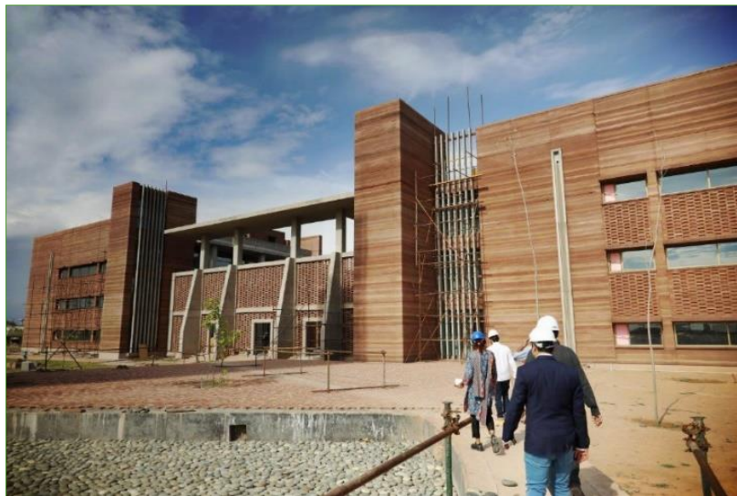
Figure 7: Rammed Earth Structure in Pakistan 36
