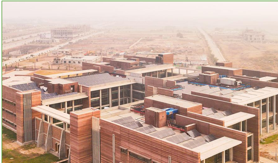
Figure 11 - PV Solar Panels, Telenor 345 Head Office
