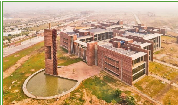
Figure 5 - Drone view of Telenor 345 Head Office
