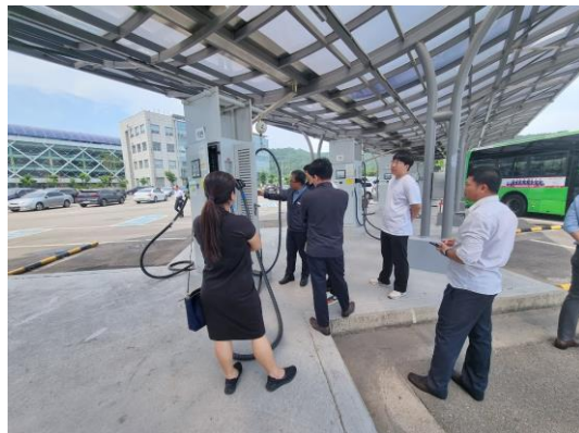
Capacity Building/Field Trip: Gangseo-gu transport garage and EV bus charging station
