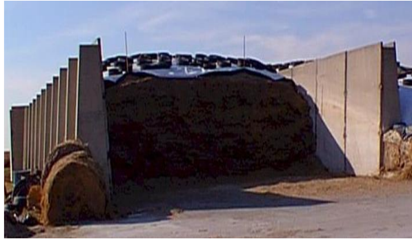
Figure 7: Bunker silo made of concrete
