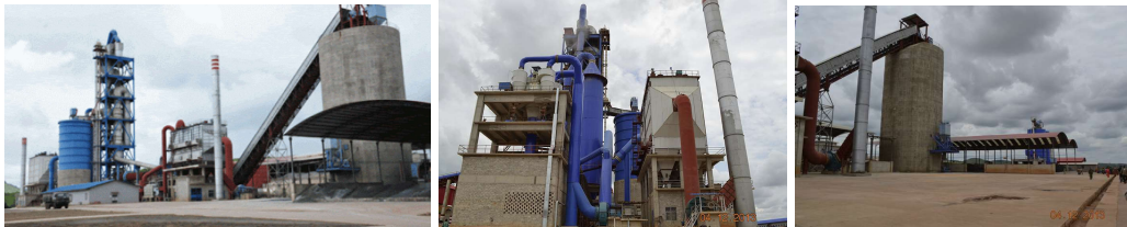
Figure 38 – FORSPAK integrated production facility near Dolisie (various views)
