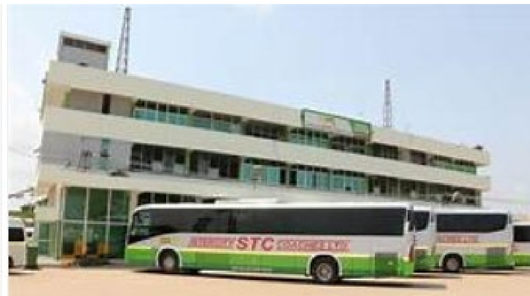
Figure 11: A pictorial view of ISTC main depot at Circle, Accra
