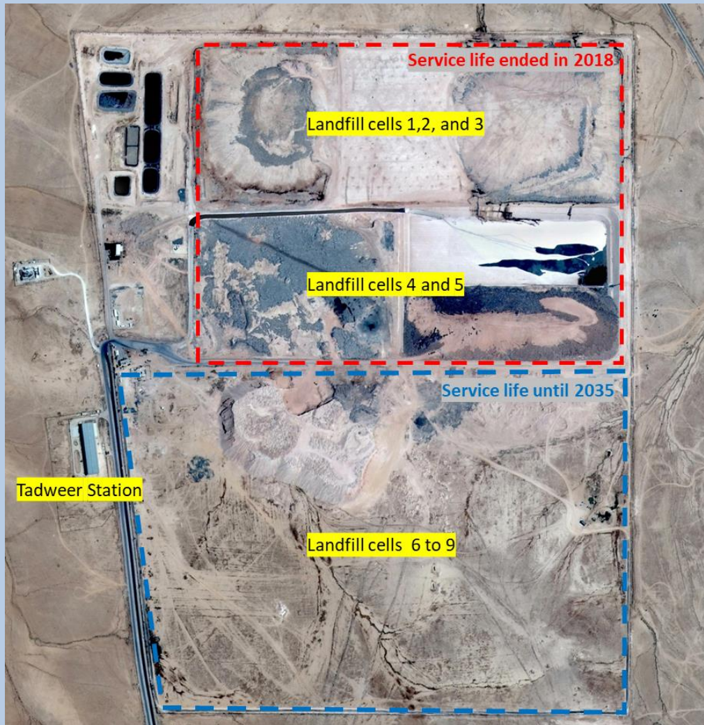
Figure 4 Ghabawi landfill and Tadweer MRF Site Close up
