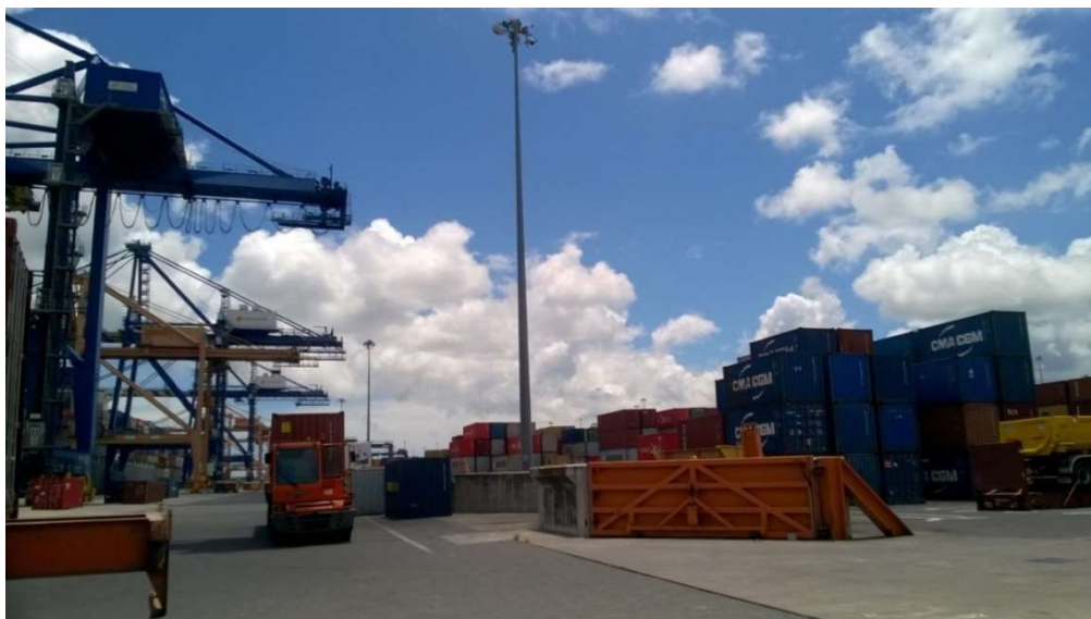
Fig. 9. View of the flood wall
