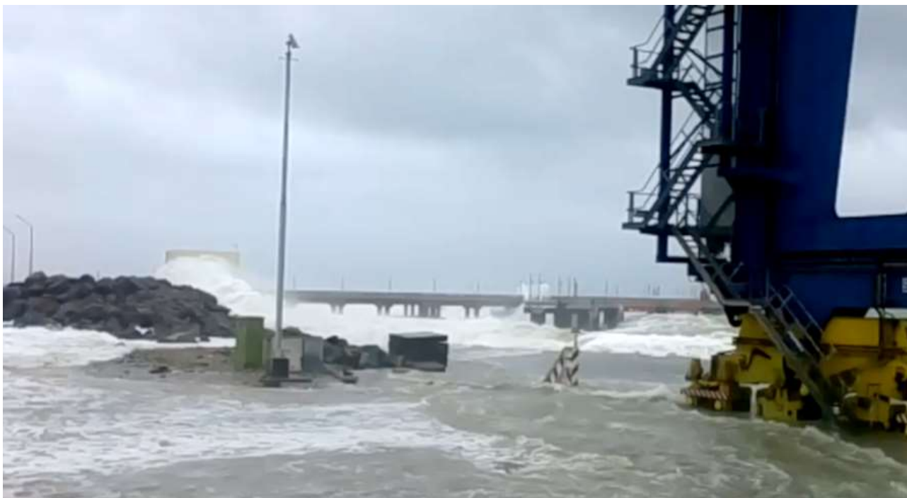
Fig. 3. Photo extracted from a video of an overtopping event at the western end of the Mauritius Container Terminal, with the oil terminal jetty in the distance (source MPA). Date and conditions are unknown.
