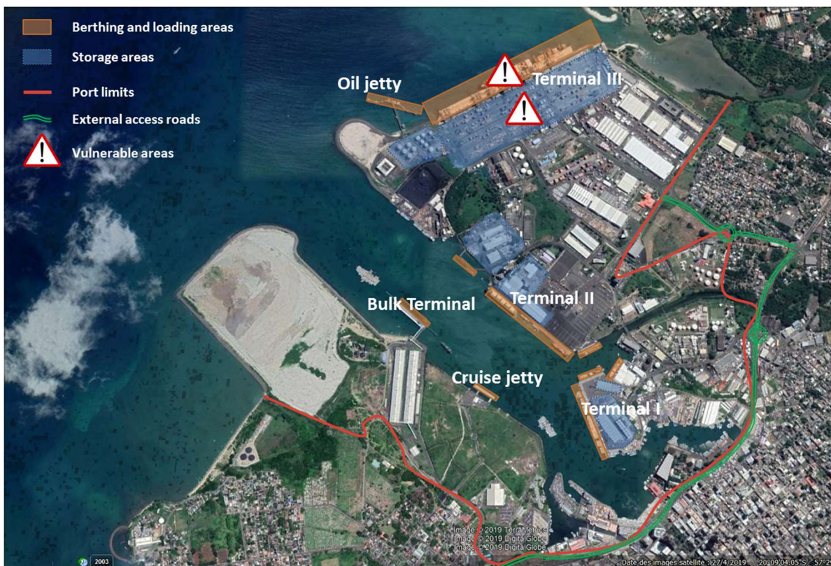
Fig. 2. Overview of the existing vulnerable areas, as identified by MPA
