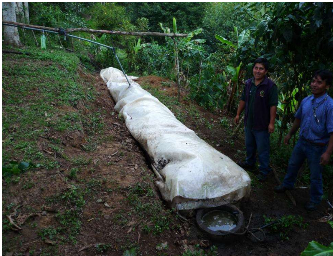
Figure 3 Tubular plastic biodigester tubular (with protective plastic cover) installed in Valle de Intag by the ACAI in 2013 (Imbabura)
