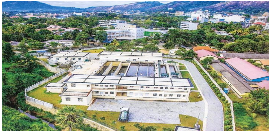
Figure 4-4) Sewerage Treatment Facility (1)
