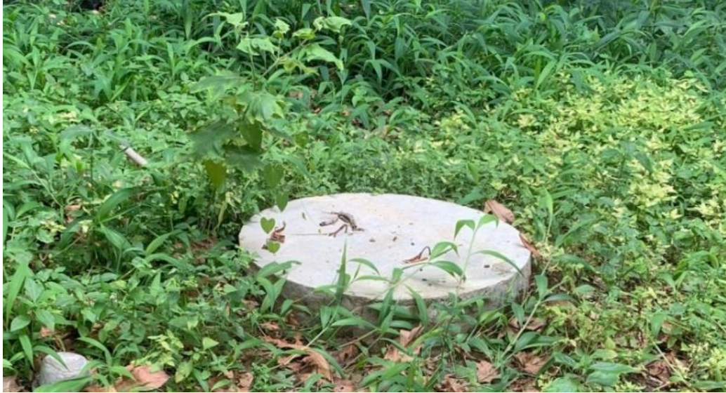
Figure 4-7) Sewerage Pit in the Garden
