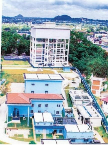
Figure 4-2) Water Treatment Plant (1)
