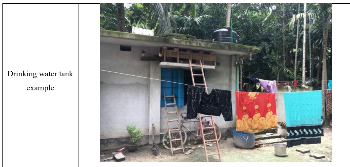
Figure 13. Drinking water facilities for households in Bagerhat district
