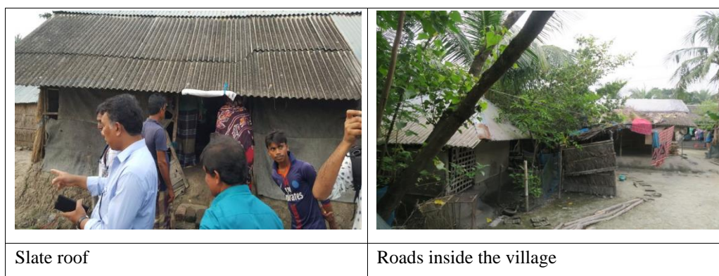
FIGURE 40 MAIN CONSTRUCTION MATERIALS IN THE VILLAGE
