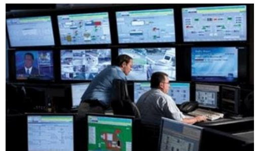
Figure 11 Data monitoring center
