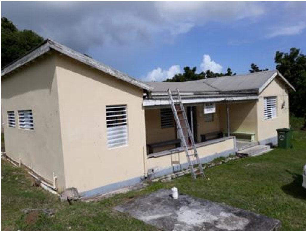
Bolans health clinic A typical small building of mortar block construction
