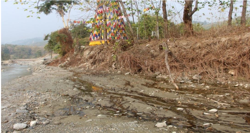
Figure 6: Highly erosive area on the left bank
