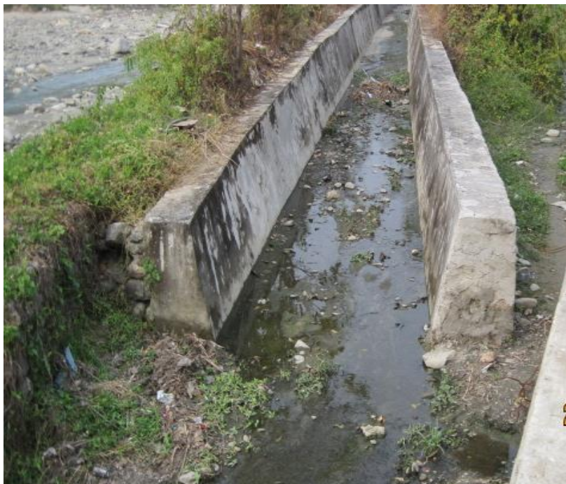
Figure 3: Outfall below the RSTA office
