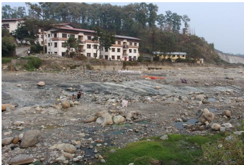
Figure 12: Vulnerable housing colony in Samdrupjongkhar
