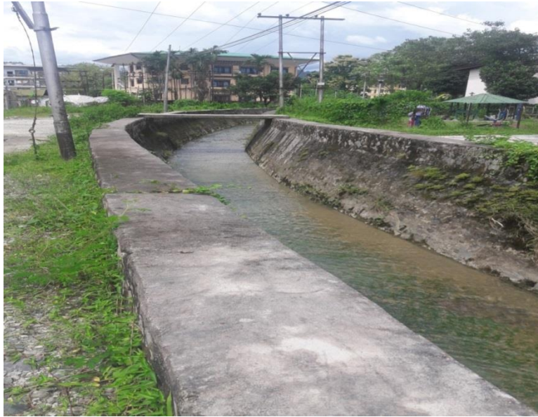
Figure 10: Storm water drain in the upper town of Samdrupjongkhar
