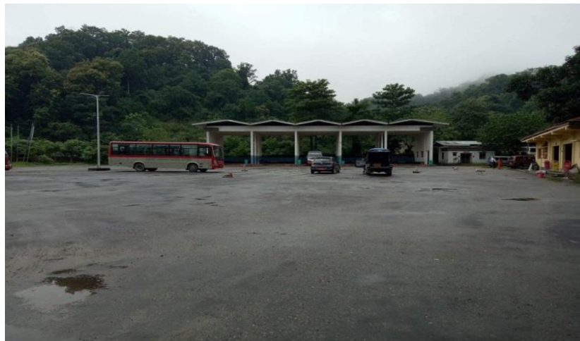
Figure 11: Bus terminal near RSTA office
