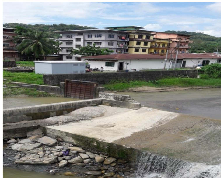
Figure 9: Weir and irrigation canal intake
