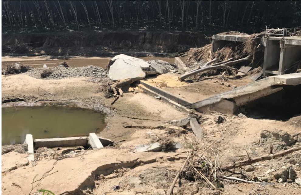
Removal of infrastructure
