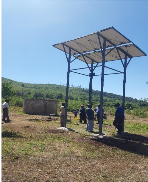
Photo 9: PV array installed to replaced mechanical wind system in Lambwe, Homabay
