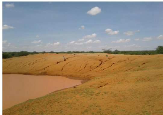
Photo 3: Siltation remain the key challenge affecting the functionality and durability of water pans
