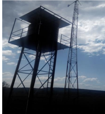
Photo 5: Hybrid system solar and small wind turbine in Baringo County. The system is not functional since the submersible pump has corroded due to high water salinity
