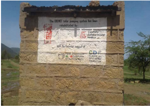
Erenet solar pumping system financed by Climate Development Foundation (CDF) and the Italian Development cooperation.
