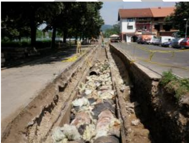
Figure 30: Pipeline Prior to Reconstruction (Trench Open, But Pipes Still Not Removed)
