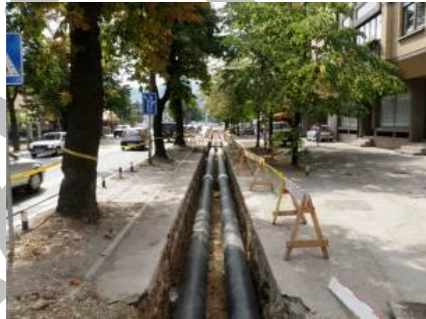
Figure 35: Pipes Laid in Soil Trench
