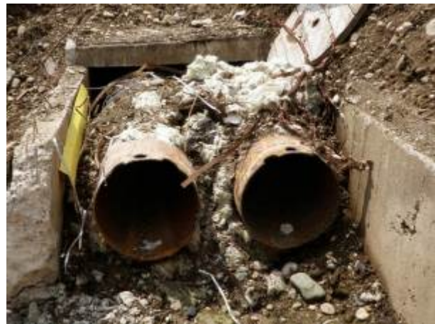
Figure 31: Trench Cross-Section (Pipeline Prior to Reconstruction)
