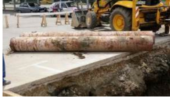
Figure 33: Part of Dismantled Pipeline
