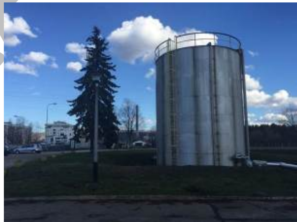
Figure 22: Aboveground HFO Tank with 2,200 m 3 and Old Thermal Insulation
