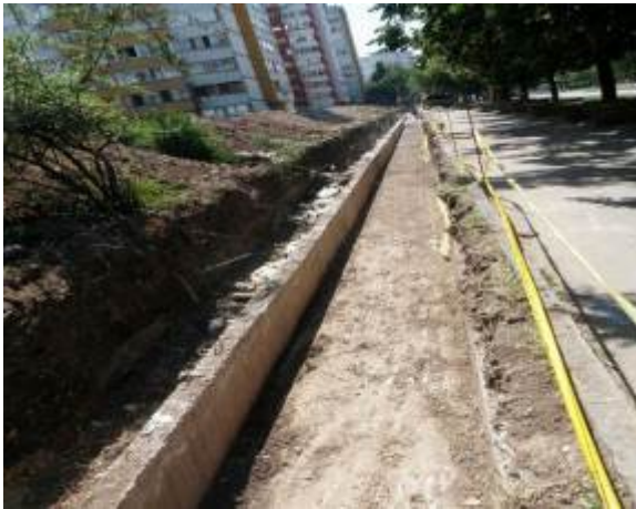
Figure 34: Concrete Trench, Cleaned and Prepared for Laying of New Pipes
