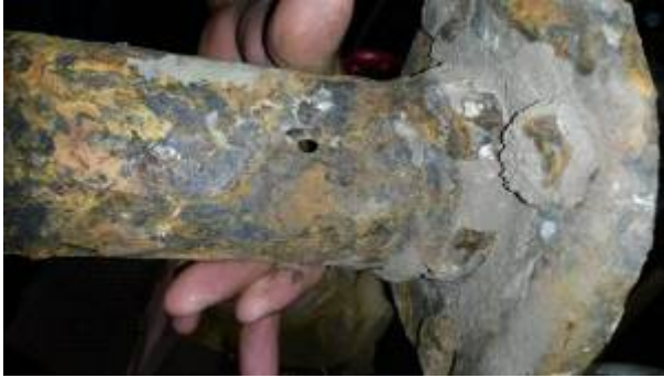
Figure 32: Part of Dismantled Pipe
