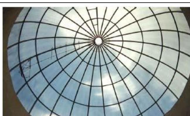
Figure 8.14. Atrium with FRP dome
