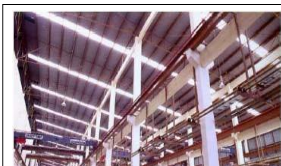
Figure 8.13. Day lighting with poly carbonated sheets
