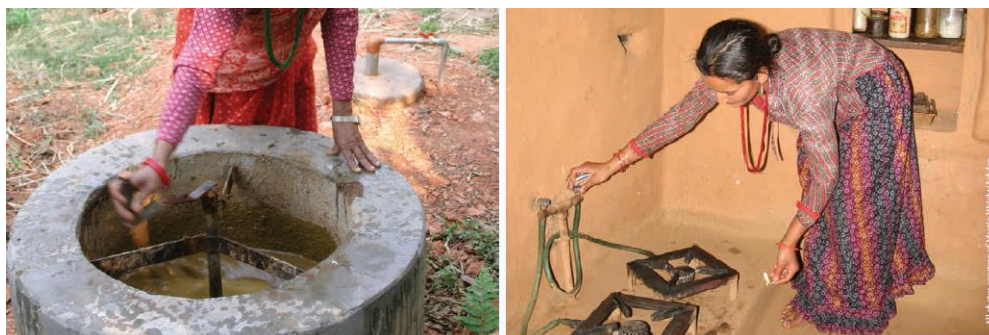
Figure 5 Domestic biogas plant and stove installed under BSP scheme
