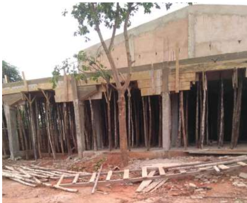
Figure 46: Different service woods in a construction site in Bobo-Dioulasso
