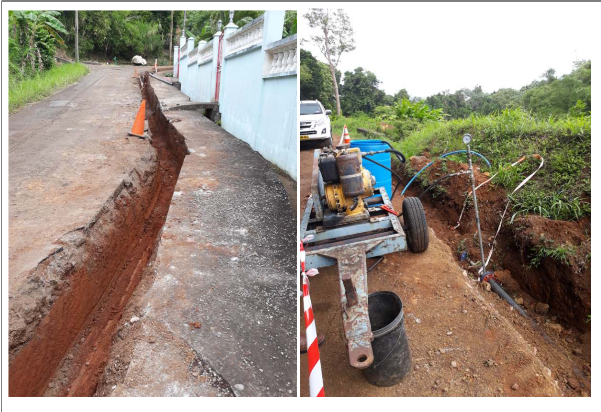
Plate 2.3 O&M activity to install the new water main asset – May 2019
