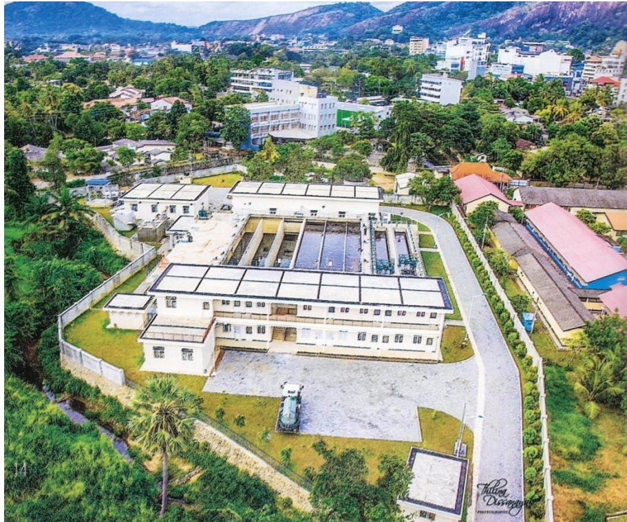
Figure 3-6) Sewerage treatment facility
