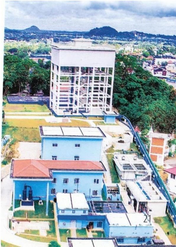
Figure 3-5) Water treatment facility
