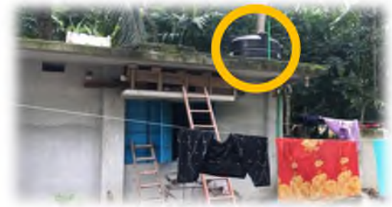
Drinking Water Tank
