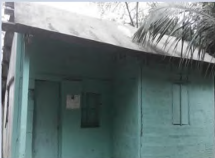
Cast-in-situ Ferro- cement Roof
