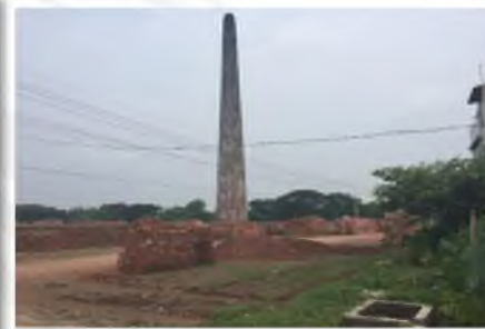
Brick Factory by use of coal fuel
