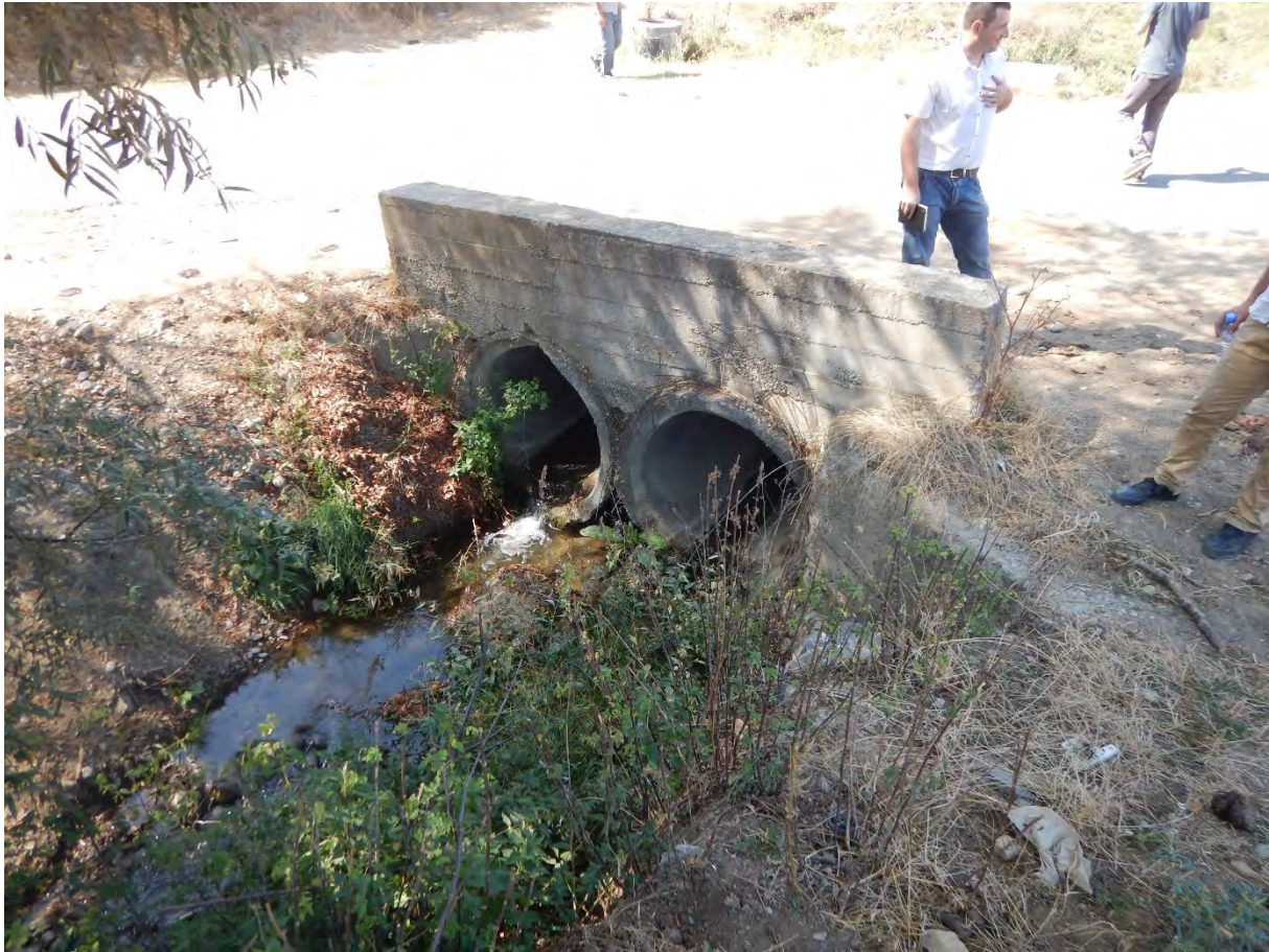
Figure 17 – Culverts in the upper Leghvtakhevi River
