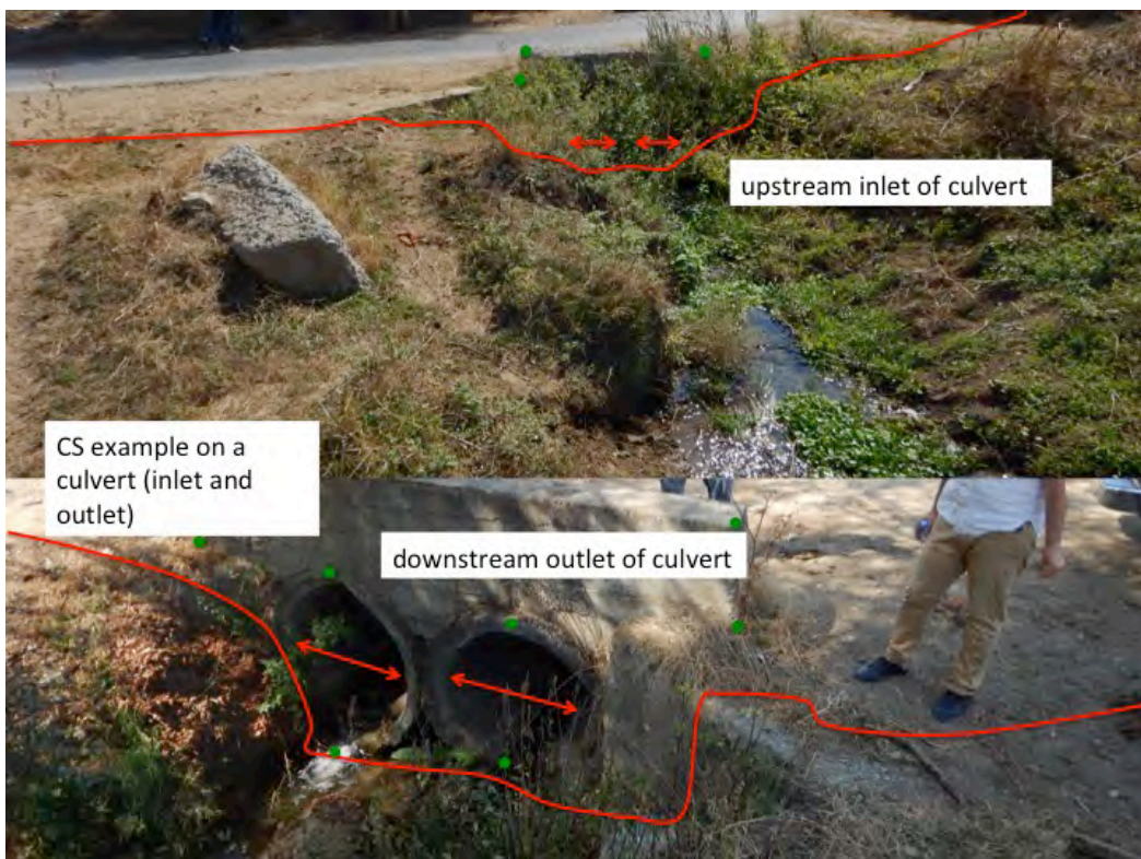
Figure 8 Cross section example on culverts
