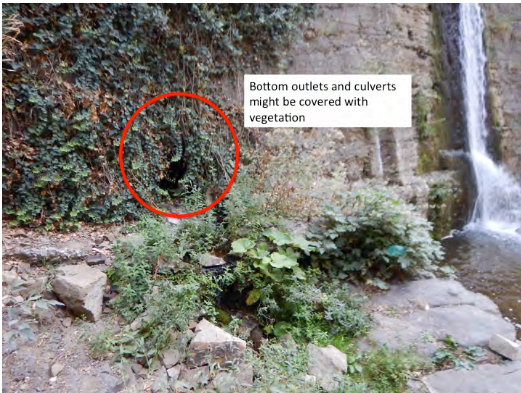
Figure 7 – Bottom outlets and culverts
