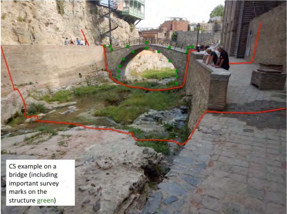
Figure 4 – Cross section example on a bridge
