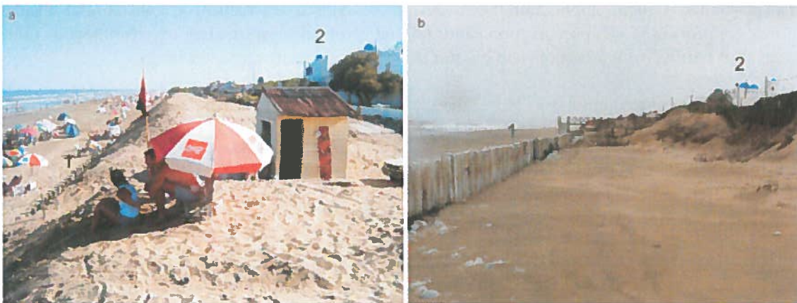
Figure 2 - Artificial recharge in the zone of high erosion in Las Toninas (Partido de la Costa): a) January 2008 – b) July 2009 (Marcomini and López, 2010)
