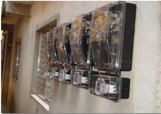
*Conventional Meters enclosed in plastic to deter tampering*
