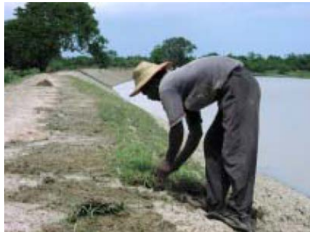
Turfing against erosion (5)
