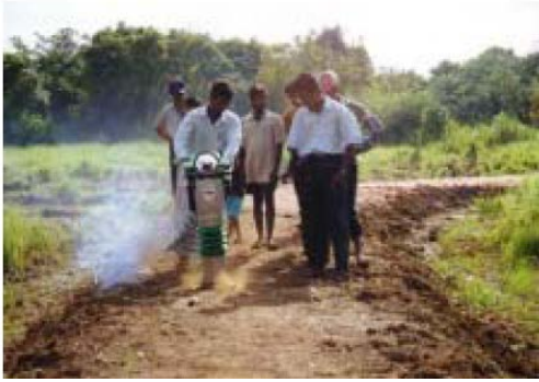
Compacting the bund (5)
