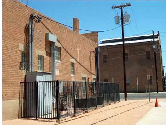
Figure 5-16. Typical commercial electrical supply panel.
