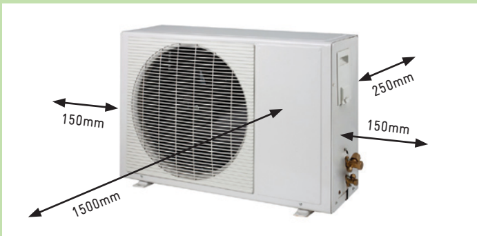
Figure 6.5 Proper Location for Outdoor Unit (ODU)
