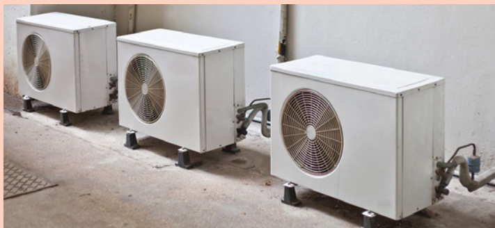
Figure 6.7 Installation of ODU
