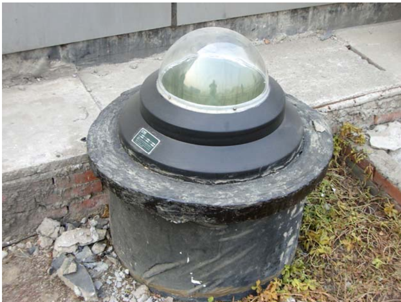
Fig.8 Light introductory system
