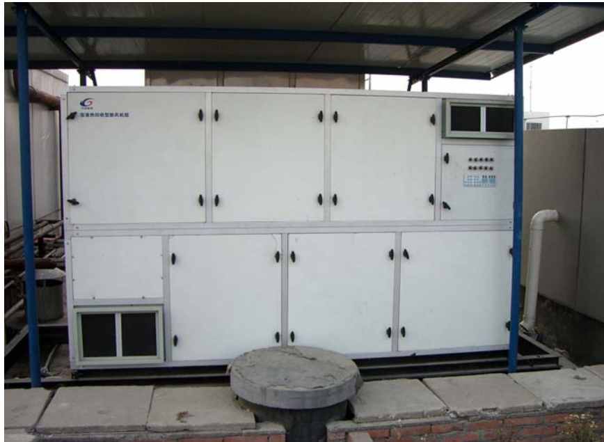
Fig.6 Dehumidification solution system
