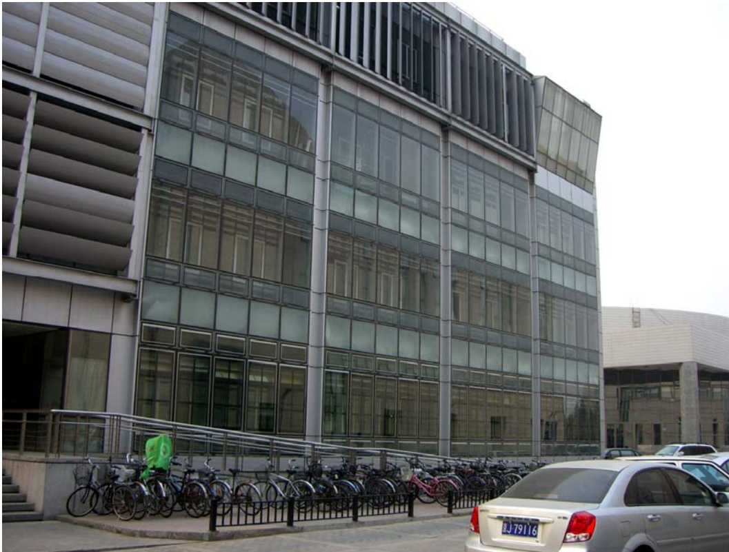
Fig.1 East façade of the building
